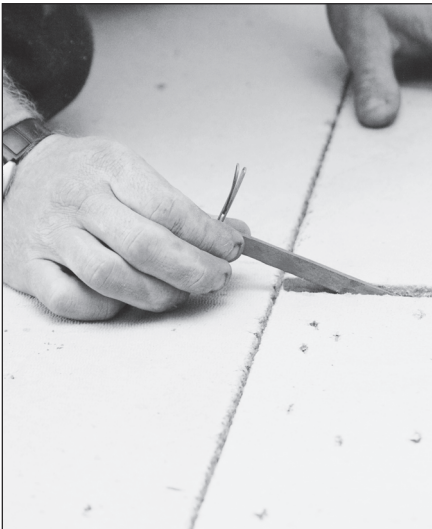
Maintain 3/16" Spacing Between Panels Read All Instructions Carefully
