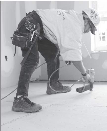
Nail and Finish Floors and Walls
